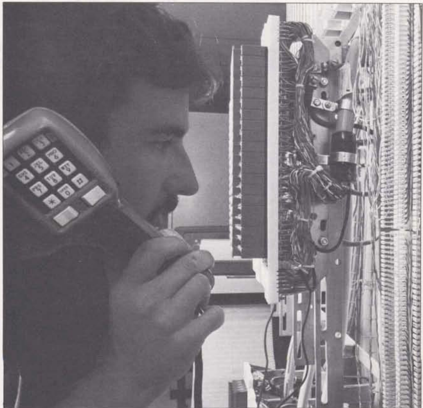
An ICSO technician with a newly-installed system.
