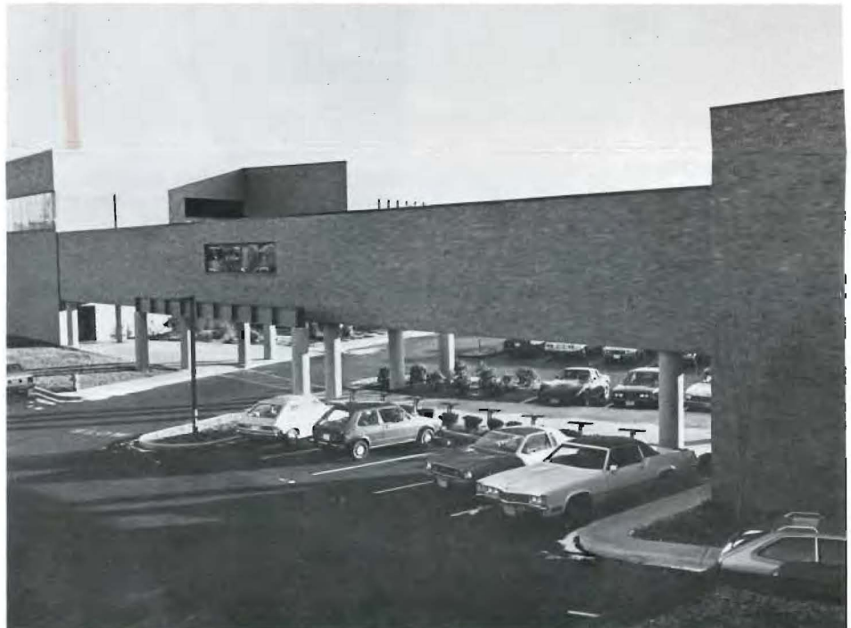
Second-story walkway links new expansion to main headquarters complex.
