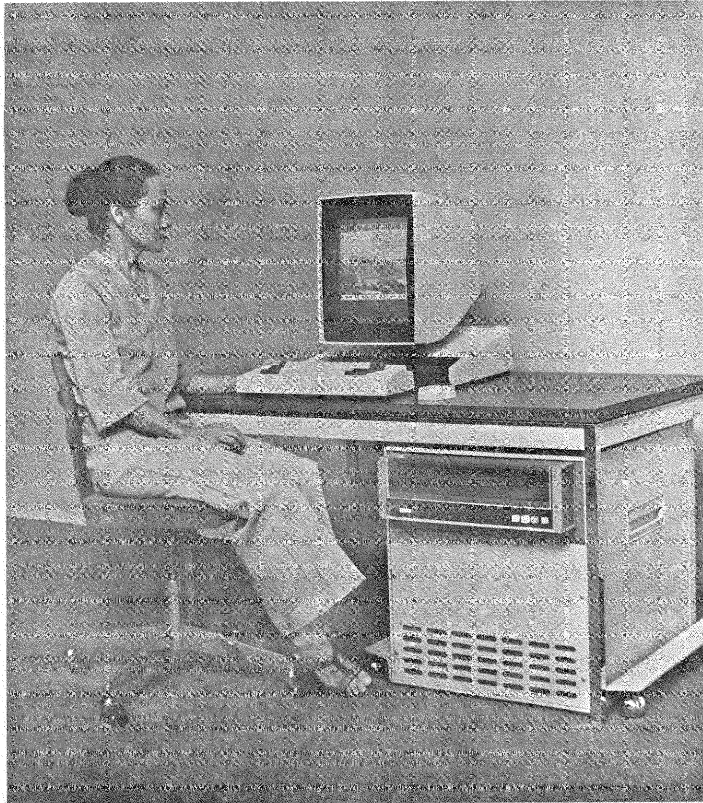
Figure 1. The Alto personal computer, showing a user at work with the display, mouse, and keyset.
