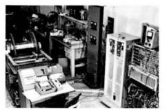
The "file-to-card" machine consists of a partially assembled disk file test bed, an 026 key punch modified for I/O service and the control electronics (against the wall). This primitive system became operable on February 10. The historic (and philosophic) first printout is shown below.
