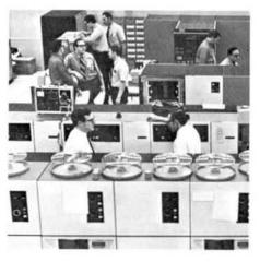
An unusual combination of San Jose's newest, biggest, and fastest disk storage products occurs when the three devices are assembled in QA's Product Measurement and Analysis area in 006 to undergo special quality tests. Being tested simultaneously by a System/370 Model 155 are the IBM 2319 (foreground), the IBM 3330 (second row) and the IBM 2305 (third unit).
