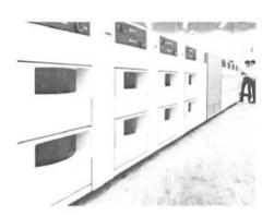
A giant among storage systems, a new 3330 Disk Storage Facility stretches out along the manufacturing floor prior to the first customer shipment from San Jose. The facility is made up of a 3830 Model 2 Control Unit and two 3333 Disk Storage and Control units (announced in August), plus six 3330 Disk Storage units.
