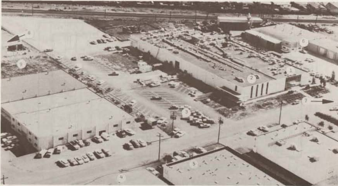
THIS AERIAL PHOTOGRAPH SHOWS MEMOREX MUCH AS IT IS TODAY. SEE STORY BELOW FOR EXPANSION HISTORY
