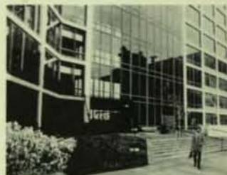
The Sherman Fairchild Building at MIT houses the School of Electrical Engineering
