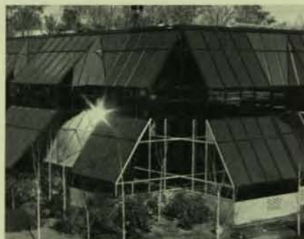
Heavy woods surround the Q-shaped center, ensuring a tranquil view out of the lab's hundreds of windows.
