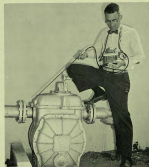
Safety engineer Mike Michols uses a "sniffer" to test for combustible gases. These devices are used to test in every area of the plant to insure that no danger spots exist.
