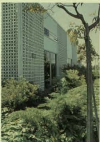
World headquarters in 1967 was one small building with a leaky roof.
