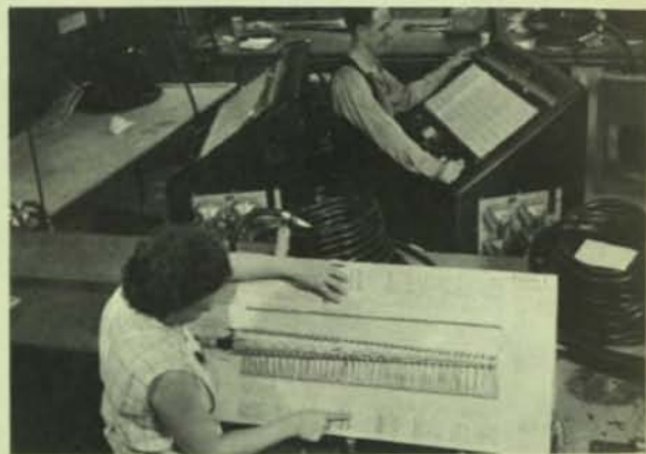
An Electronic Circuit Analyzer checks out a cable assembly fast and accurately.
