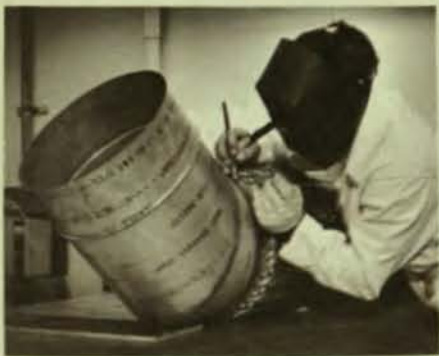
Welding segmented section of liquid oxygen fuel line used on Titan and Atlas missiles. Exact requirements demand that welders performing such operations be U. S. Government certified.
