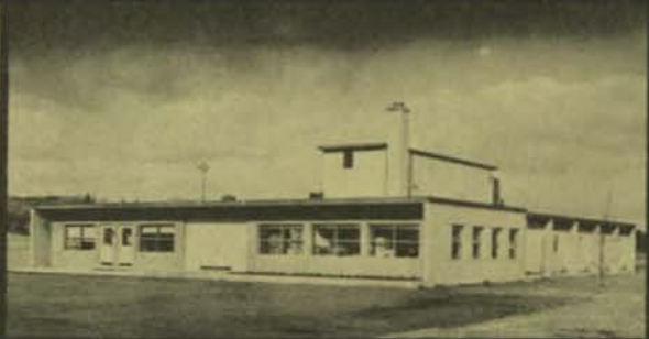
Left—Offices and Plant Graphic Equipment Division, Plainview, L. I., N. Y. 58,500 square feet
