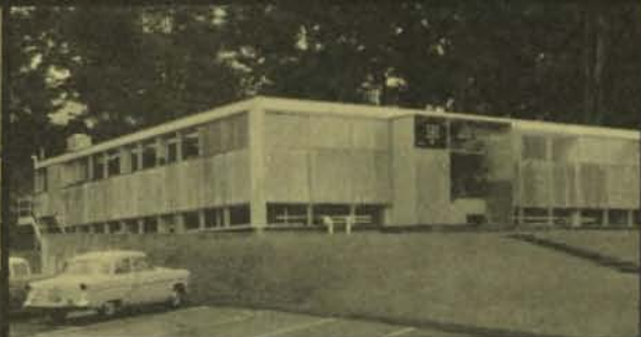
Left—Engineering Building, Defense Products Division, Syosset, L. I., N. Y. 58,500 square feet
