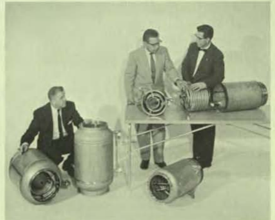
Heat exchangers used in Atlas and other ICBM's are shown above. Similar units were used in Mercury Man-in-Space project.
