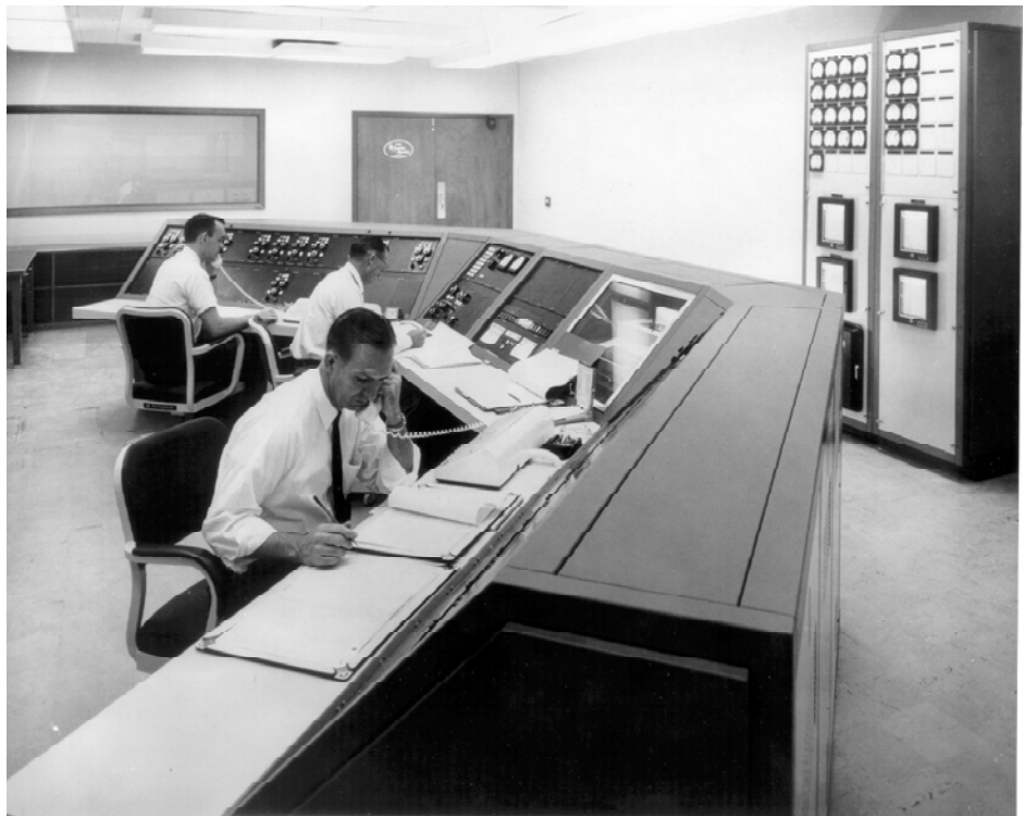
Right - Arizona Public Service and Salt River Project dispatchers at the ADDAPS console in Phoenix. The Prodac-580 performed economic calculations and controlled all the electricity generated in the state of Arizona.
