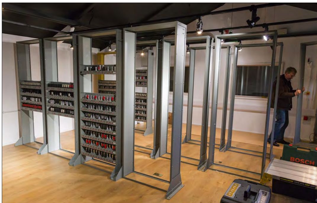
Figure 4: EDSAC gallery and racks under construction
