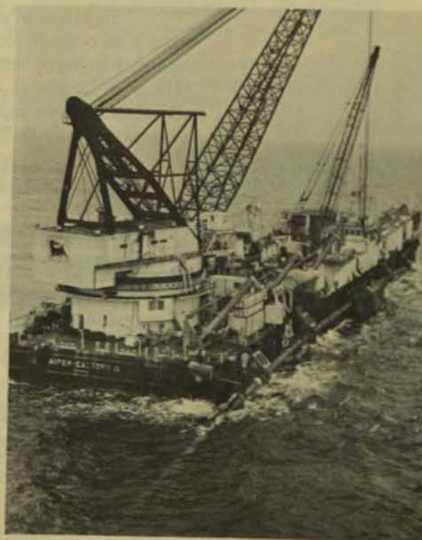
This barge linked the pipeline from BP's North Sea field.
