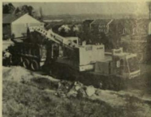
A new Gradall G-660 excavator assists with street repairs in Timonium, Maryland. The contractor used versatile Gradall excavators for initial land clearing and then to build streets, storm drains, sewers and sidewalks.
