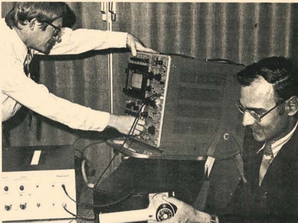
PHOTO'S BOB MCCONNELL, LEFT, AND TID'S NORM STAUFFER Measuring the color output of a Strobolar with new multi-channel spectrometer.
