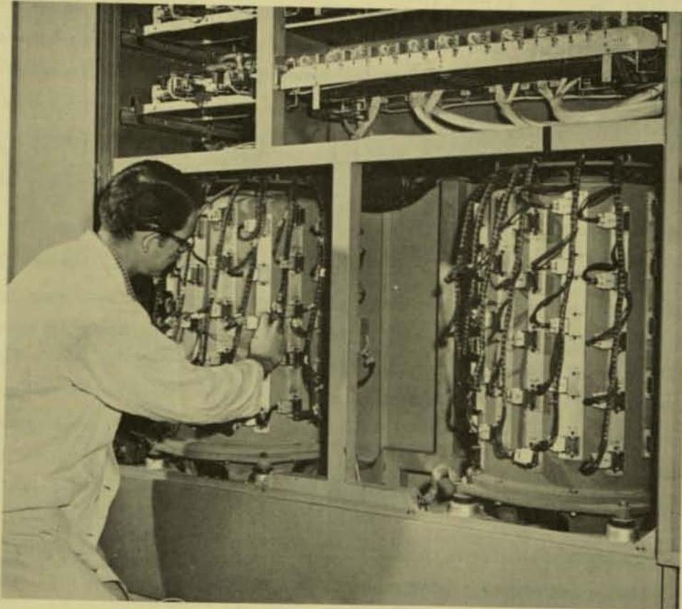
ERMA's magnetic drums are contained within these vertical cylinders. The drums store current balance, stop-payment and hold information for future use.
