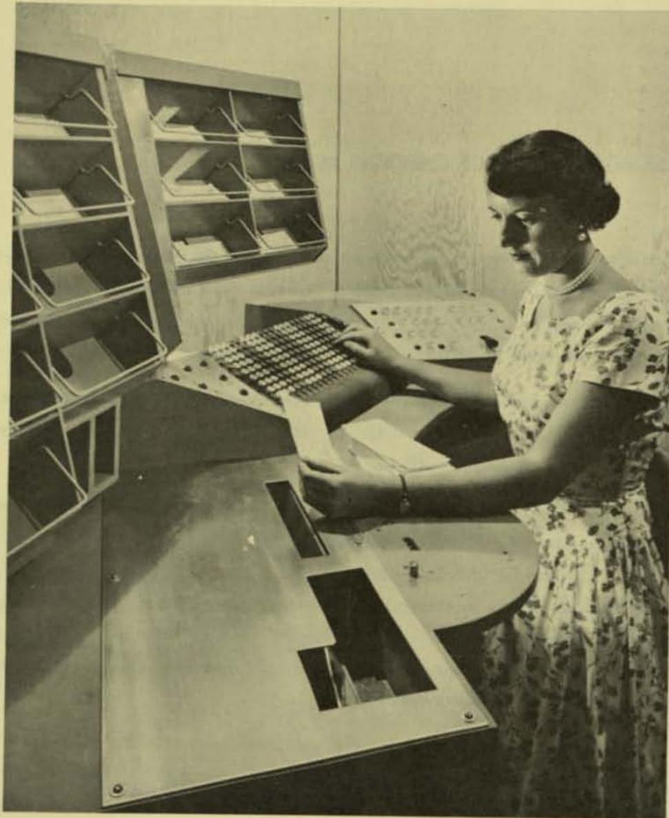
Operator at the input console. The amount of deposit or withdrawal is punched on the keyboard, the check or deposit slip is dropped in the automatic reader, then ERMA's work cycle begins.
