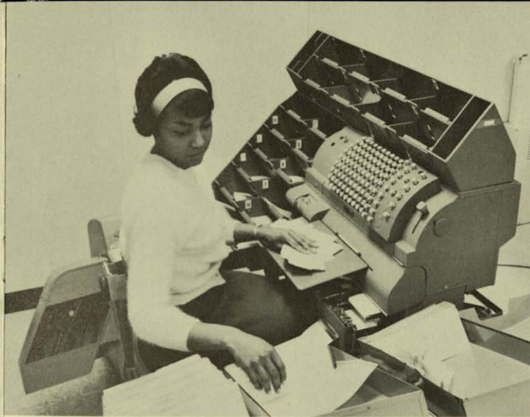
Amount Encoder—an attachment to the N.C.R. Proof Machine, illustrated here. We call this post-printing.
