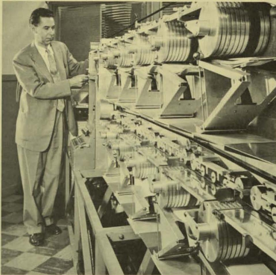
Another view of the check sorter which sorts by account number. Each bundle of checks must be passed through the machine five times (once for each digit). The checks travel at the rate of 150 inches per second through the sorter.
