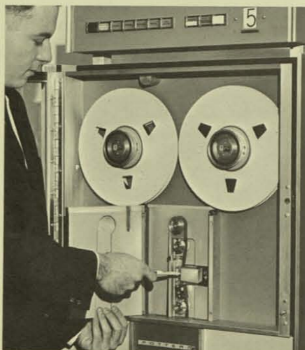
Figure 5. Automatic Tape Loading
