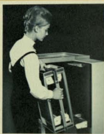
Places Cartridge on Loading Carriage.
