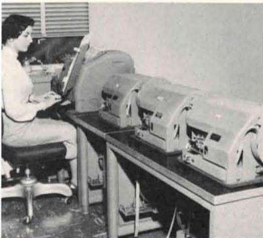
**DISTRICT** sales office operator, in creating invoice on teleprinter, puts data for stock control and other purposes into tapes from reperforators. Tapes are converted into tabulating cards.
