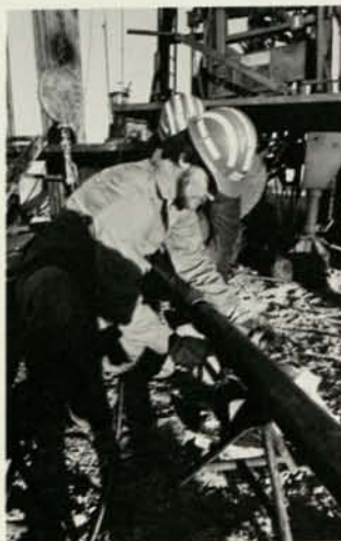
Rigging up a logging tool on location outside Midland, Texas.
