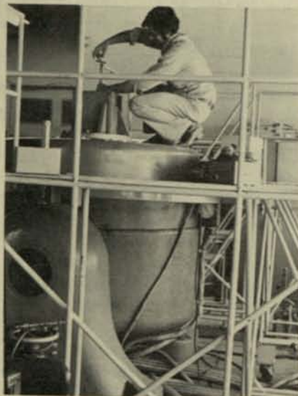
A room-size vibration machine shakes down products before they are delivered to the customer.
