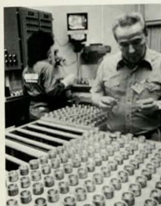
Checking shaped charges used in well development at the Schlumberger Perforating Center in Rosharon, Texas.
