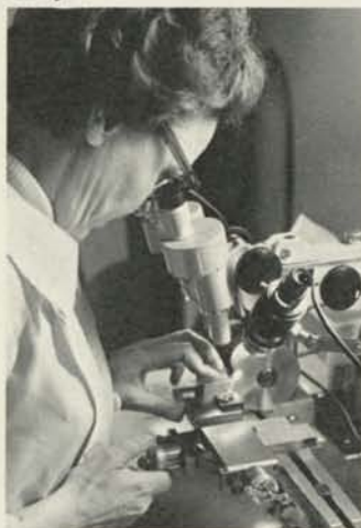
Machinist Marge Peterson laps a bonding tool on a jeweler's lathe.
