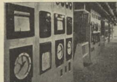
110 Electronik Instruments measure and control temperatures at I.C.I. "Terylene" Plant—Wilton, Yorkshire.
