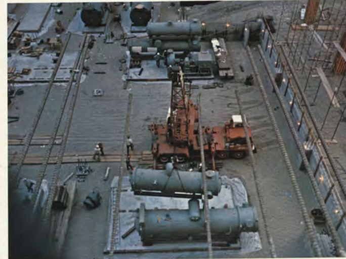
Atlantic Richfield Plaza/(Placing centrifugal refrigeration units) Los Angeles, Calif.; Albert C. Martin and Associates, Architect; W. A. Di Giacomo and Associates, Mechanical Engineer; Turner and McKee Construction Company, General Contractor; completion scheduled, 1971.
