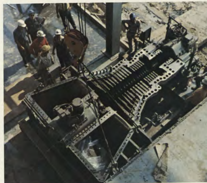
Steam Turbine Placement in Worthington Combined Cycle Power Plant/Lake Charles, Louisiana.
