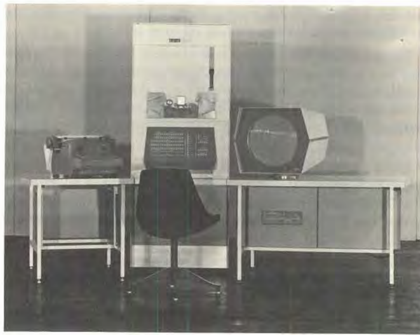
DIGITAL'S EARLIEST COMPUTERS WERE A SIGNIFICANT DEPARTURE FROM SYSTEMS OF THAT ERA. THEY WERE PHYSICALLY SMALL, INTERACTED DIRECTLY WITH THE USER THROUGH A VIDEO OR KEYBOARD TERMINAL, AND BROKE THE MILLION DOLLAR PRICE BARRIER
