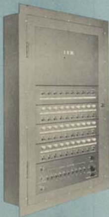
Central Operations Panel
