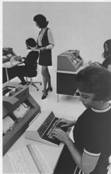
▲ The IBM 129 Card Data Recorder has a monolithic-circuit memory that helps speed punching of familiar 80-column cards for computers and other business machines.
