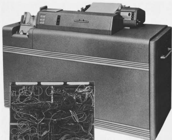
▲ The IBM 407 had punched card input on the left and printer in the center top. This was the last of the electromechanical accounting machines.
