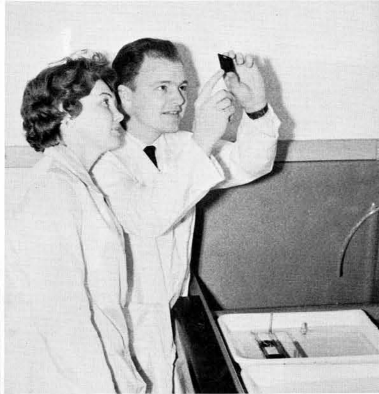
In one of the lab's photographic darkrooms Supervisor Dick Robinson and Assembler Margaret Burroughs check the same mask after it has been reduced photographically to its final dimensions. Any impurity, even a particle of dust too small for the eye to see, can ruin the tiny masks. Hence lab personnel and visitors must change into "clean" clothes and undergo a vacuum cleaning before entering this section of the lab.
