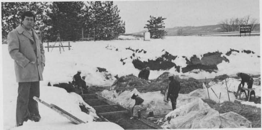
Frank Zupan checks on construction progress.
