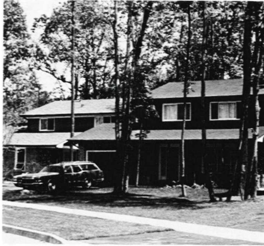
TORONTO NEW TOWN developer, Cadillac Fairview Corp., Ltd., Canada's largest integrated real estate development company, uses Tymshare's FOCUS system for planning and analyzing land use yield in 7800-acre Erin Mills new community project. Residential areas like this will house some 170,000 people.
