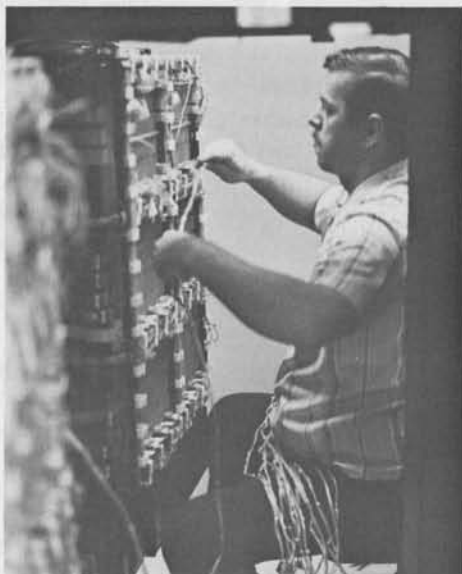
Chuck Cochran, FSE, Portland, installs tri- leads from the Memorex 6258 to the IBM 370/158.
