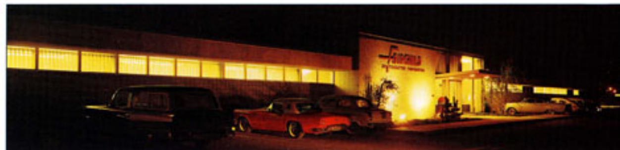
Fairchild's main office and transistor manufacturing plant, occupying 68,000 square feet in Mountain View, California. This expanded facility was necessitated by production requirements less than one year after Fairchild's first product announcement. Further expansion of this facility is planned for early 1961.
