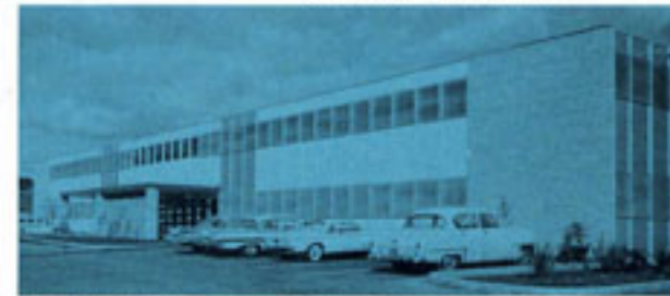
Fairchild's 52,000 square foot diode plant in San Rafael, California, was occupied in November 1960.
