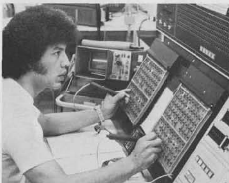
Test Technician Art Cortez observes the readout of Memorex digital tester while troubleshooting a 3671 PCB. The tester was built in-house by the test engineering department.
