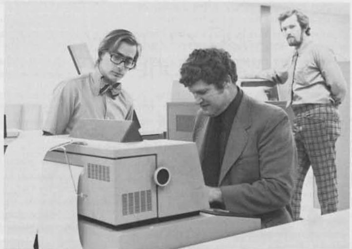
Attached to a host computer, the 3672 Disc Storage Control Unit is tested in various customer applications in different operating systems. Above (l to r) Ken Holly, Staff Engineer, Mills Qualls, Engineer, and Ulf Peter Motzfeldt, Staff Engineer, perform this unique customer level testing to insure the new 3672 operates satisfactorily in any customer environment.
