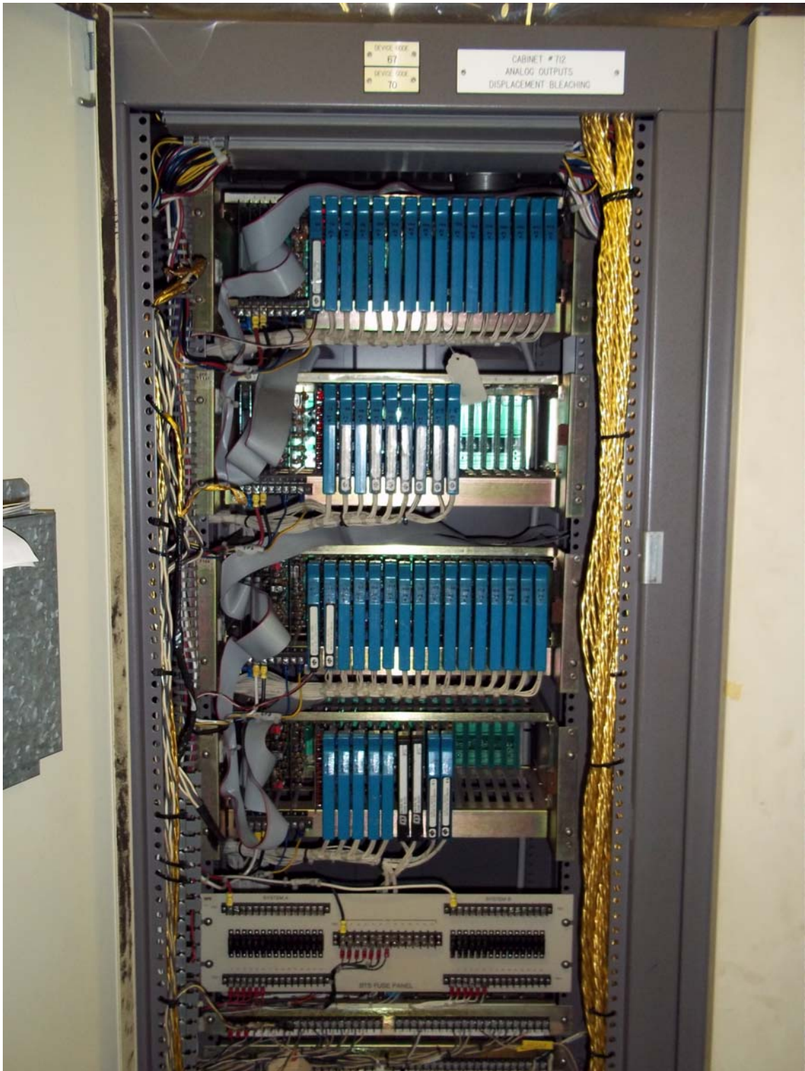
This photo shows a bay of AO cards and their connectors. Note the identical cards in identical chassis. The top two chassis are connected to the A computer; the bottom two are connected to the B computer.
