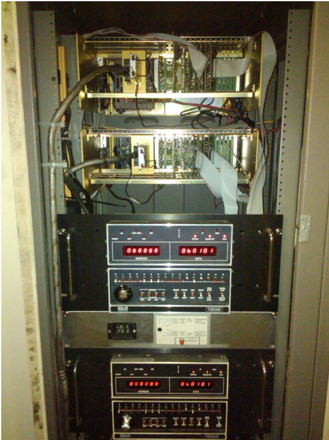
The upper part of the same bay shows the two front panels better. Above them are the two IOBCs, which interface the ROLMs to the Computer Products I/O gear.
