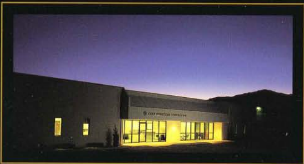
Printed Circuit Board Facility.
