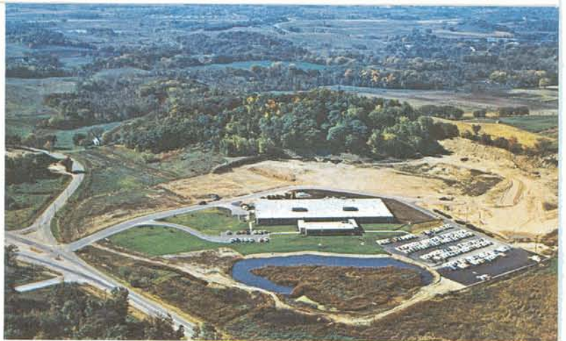
This new, ultra-modern facility was built specifically for the design and production of TEC-LITE Indicator Devices, Digital Readouts and precision electronic subassemblies. Here, DATA●PANEL was conceived and is now produced. Photos are: 1) view of 52,200 square foot fully climatized administrative offices and plant; 2) a production area with high level lighting and spacious, efficient layout; 3) TEC-LITE inspection area where specially built test instruments duplicate in-system electrical conditions.
