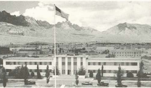
ROCKETRY'S HUB—Landmarks for White Sands Missile Range and its more than $37.5 million a year payroll are this new, active headquarters building, the 110-foot flagpole fronting it, and the towering Organ Mountains in the background. From the office of the Commanding General come the administrative orders affecting more than 9,000 military and civilian personnel at work at White Sands Missile Range on the various missile projects.
