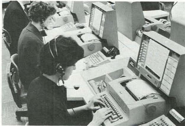
↑ SABRE, the airline reservation system, was the first large commercial computer network that operated on-line in real-time. That is, changes in schedules and reservations were recorded as they occurred. SABRE significantly reduced the time needed to make reservations. SABRE was developed by IBM for American Airlines after six years of joint research. It went into operation in 1962.
