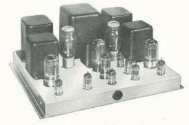
This power supply is a highly stable unit which features voltage regulation by a single 5651 tube. It is well rated for its use.
