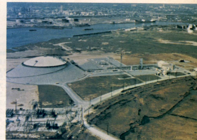
Texas Eastern Transmission Corp.'s liquefied natural gas (LNG) storage facility at Staten Island, New York, is of prestressed concrete and represents a first of its kind for storage of fluids at cryogenic temperature.
