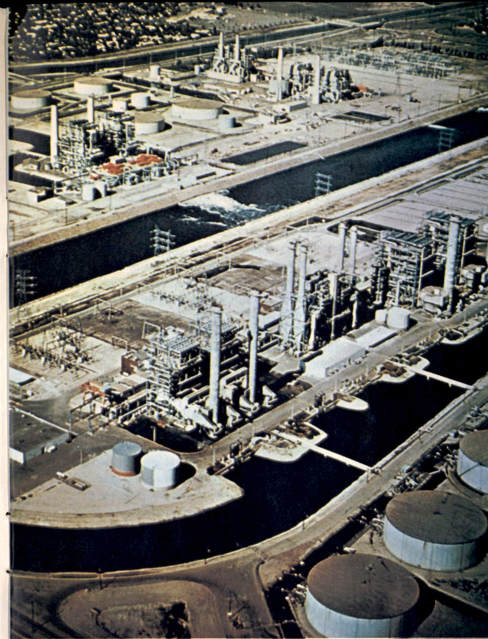
Vast complex of power stations built to supply the energy-thirsty Los Angeles area. Twelve fossil-fueled boilers with a combined capacity of 3 million kw are located in a 3-square mile area.
