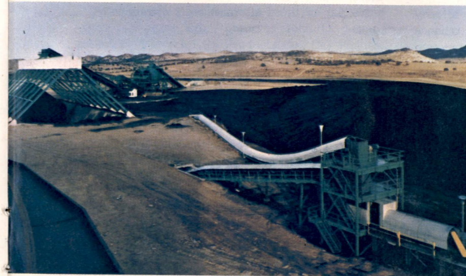
Coal preparation, storage, and conveying facilities at Peabody Coal Co.'s Black Mesa mine. From this point, coal is transported by slurry pipeline 275 miles to the Mohave generating station at Davis Dam in Nevada.
