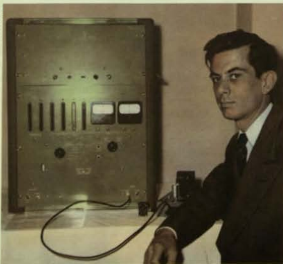
In 1951, Al Bagley's development of HP's new 524A high-speed frequency counter reduced the time needed to measure high frequencies from minutes to seconds.
