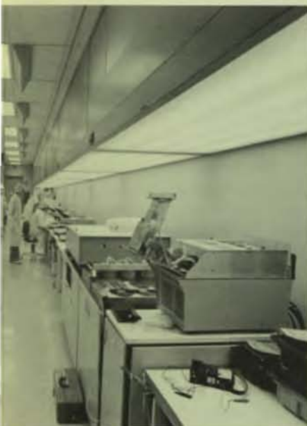
3. Fab areas are entered through automatic sliding doors, which prevent the vacuum created by regular hinged doors.
