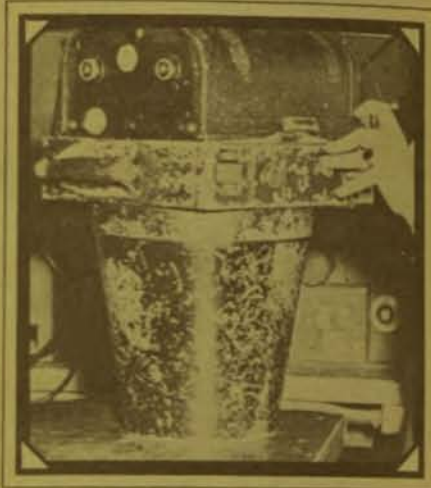
Not exactly as easy to handle as today's pocket camera, the early aerial camera worked because it combined a long enough focal length with Fairchild's new shutter, capable of a shutter speed of 1/1000 of a second.
