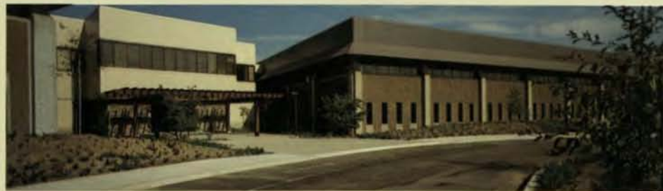
Tandem headquarters facilities in California more than doubled during fiscal 1980 with the addition of 165,000 square feet of manufacturing, marketing, and research and development space. Elsewhere during the year Tandem opened 16 new offices and 10 additional educational centers for customer training.
