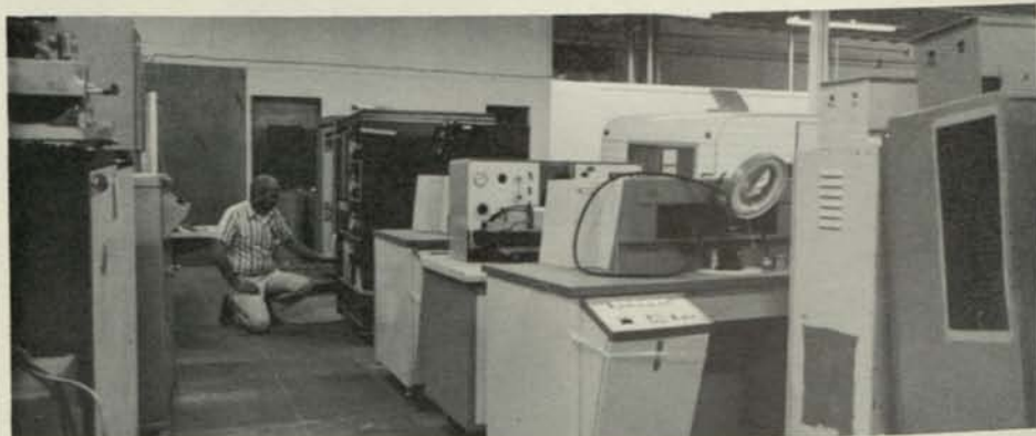
Jim Green surveys the larger pieces of equipment for defects before entering them into the shopping list for supervisors and managers.
