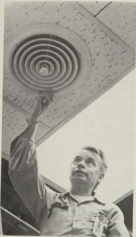
Repairing a broken air conditioning unit in Building 7 is Fred Bloom.
