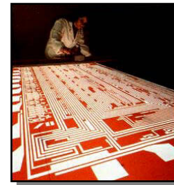
MUX layout with gate mask programmability. (No CAD) Voila, the semiconductor ROM!
