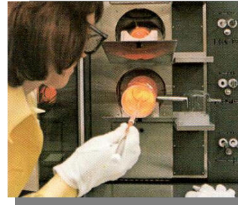
Installed wafer fab ($300K)
