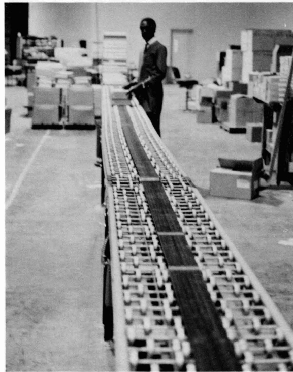
Conveyor belts installed at the Manufacturing plant speed the packaging and shipping of products, according to Mel Holmes.
