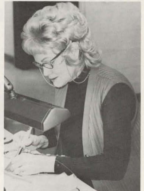
Lorraine Brame, a senior sub-assembler, solders a printed circuit board.
