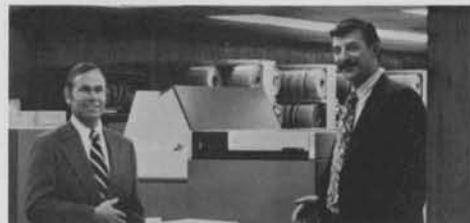
At American Motors Corporation's Data Center, the first Memorex 3672 is installed and running smoothly. Pictured left to right are happy Memorex Salesman Tom Koch and AMC's Data Center Manager Bob Alexy.
