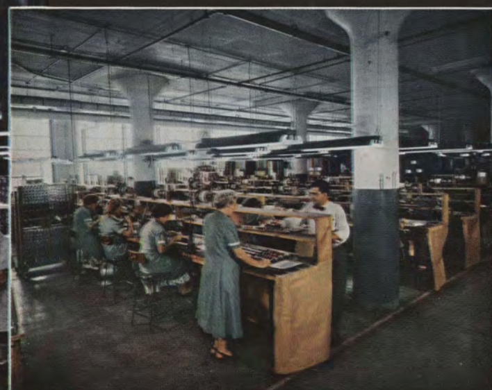
Key to serviceability of Univac is its many removable service units, known as "chassis." These are fitted into sections, three of which form each bay. Experience has proved that women are best for this precision assembly.
