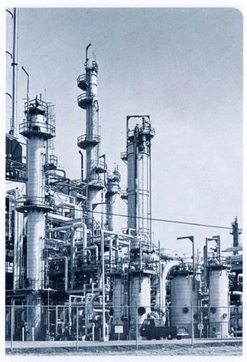
PETROLEUM Refinery information and oil movement systems, cracking plants, and crude oil units are all key refinery applications for process computers. Other applications include product blending, reformers, alkylation units, and lubricants of wax plants. Computers have also been successfully applied to on-shore and off-shore production, crude and production pipe lines and truck terminals.
